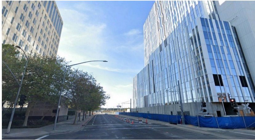
Figure 11 Viewpoint 2 from 6th and H Street Intersection (looking west)
