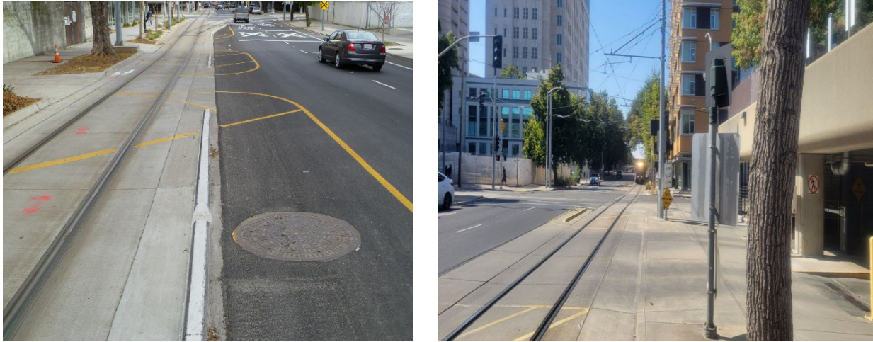
Figure 8 Photographs along H Street of Typical Light Rail Embedded Track on Concrete
